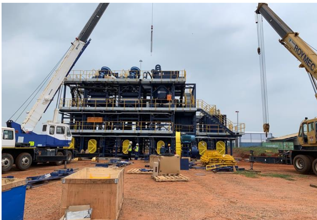
TRP being assembled for pre-delivery commissioning
