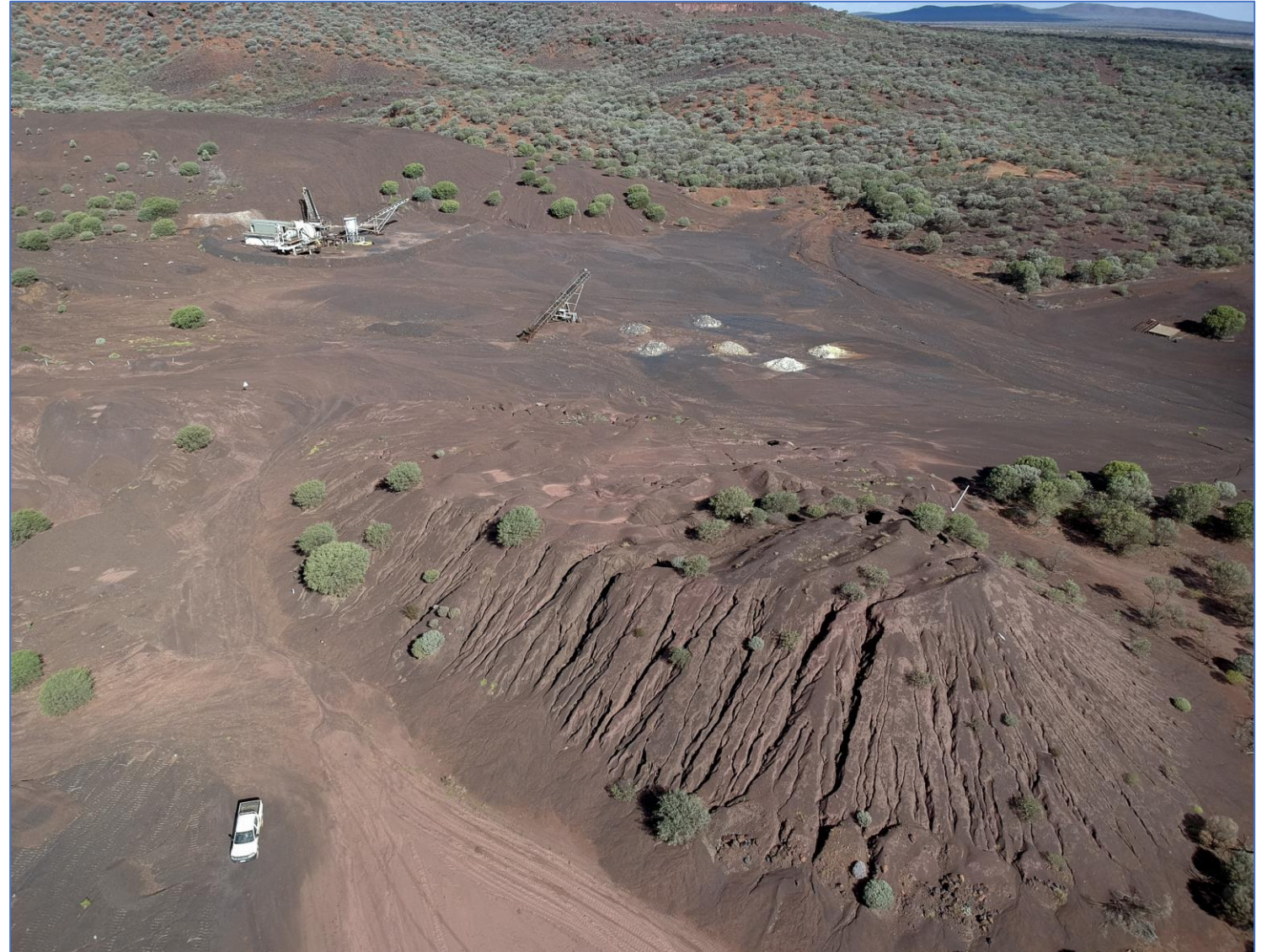
View of old DMS plant and manganiferous stockpiles from previous mining operations.
